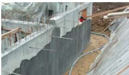
VANDEX CEMELAST as external waterproofing.
