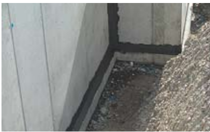
VANDEX CONSTRUCTION JOINT TAPE external application at horizontal and vertical construction joints.
